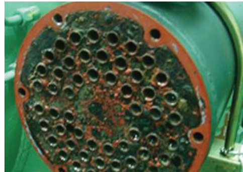
After 6 Months of Installation of EST
