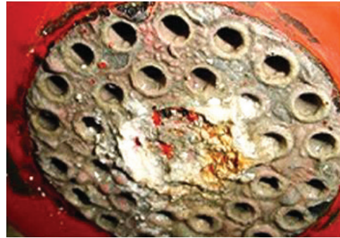
Before Installation of EST
