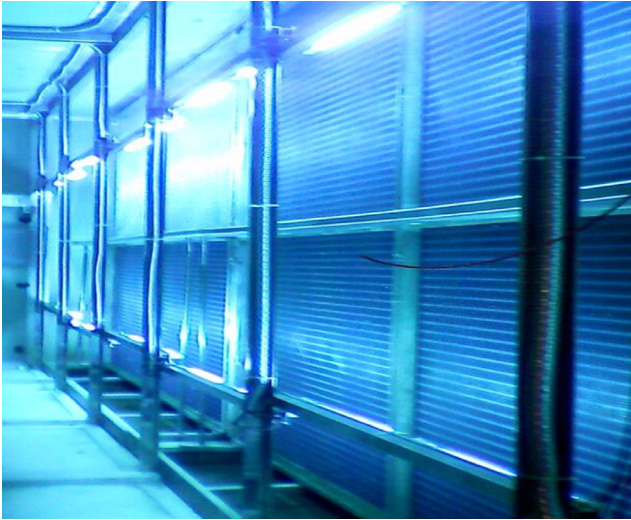
Coil-o-Care - UVC Lamp Assembly Arrangement for AHU Coil Cleaning
